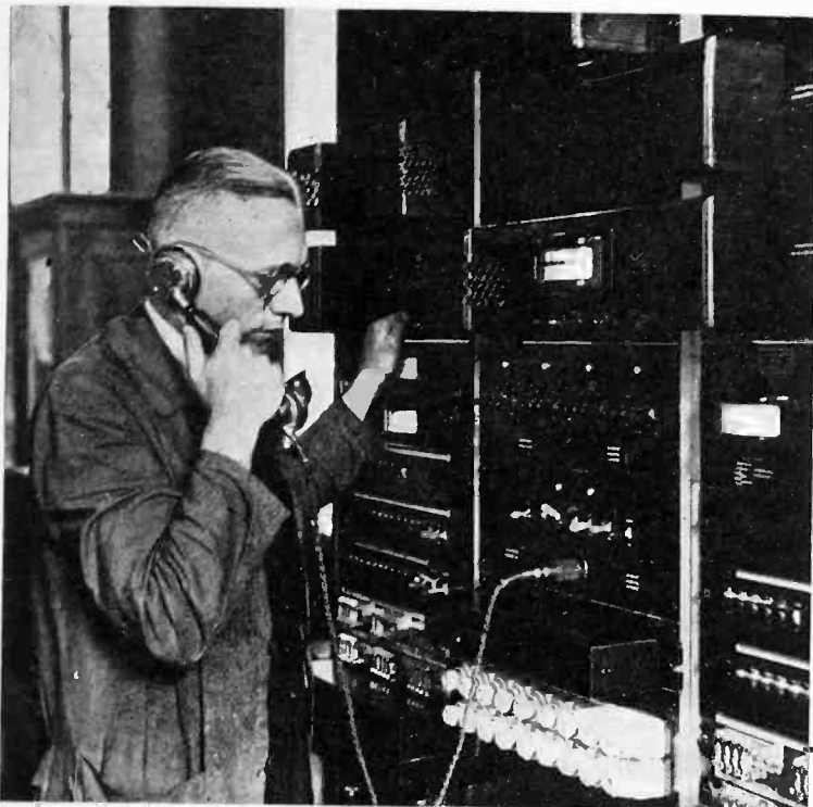
The Berlin-London facsimile circuit. Interior of transmitting room of the German Reichspost service which works co-operatively with the British Post Office, Paris, and Rome, by wire
